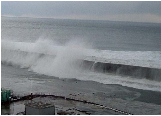
Figure 3: Sea wall breach.
